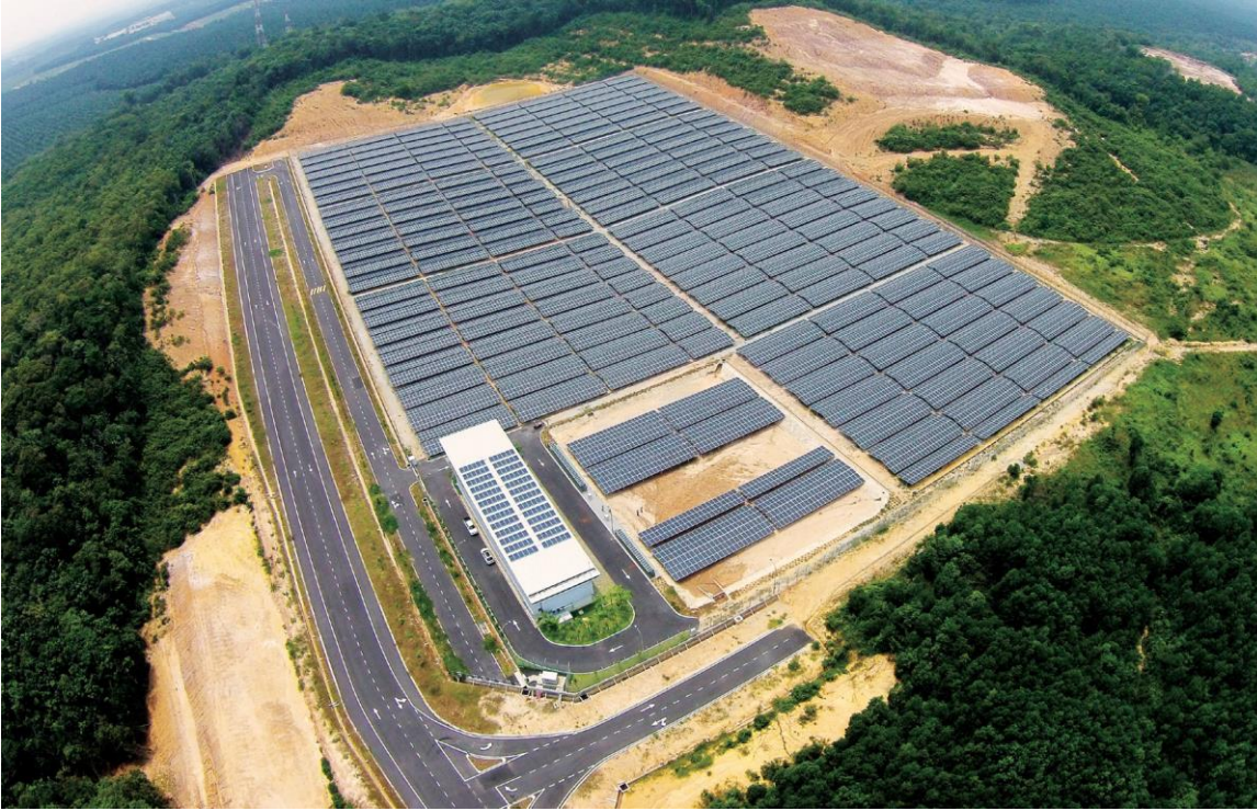
Example solar power facility - Hang Tuah Jaya, Malaysia.
